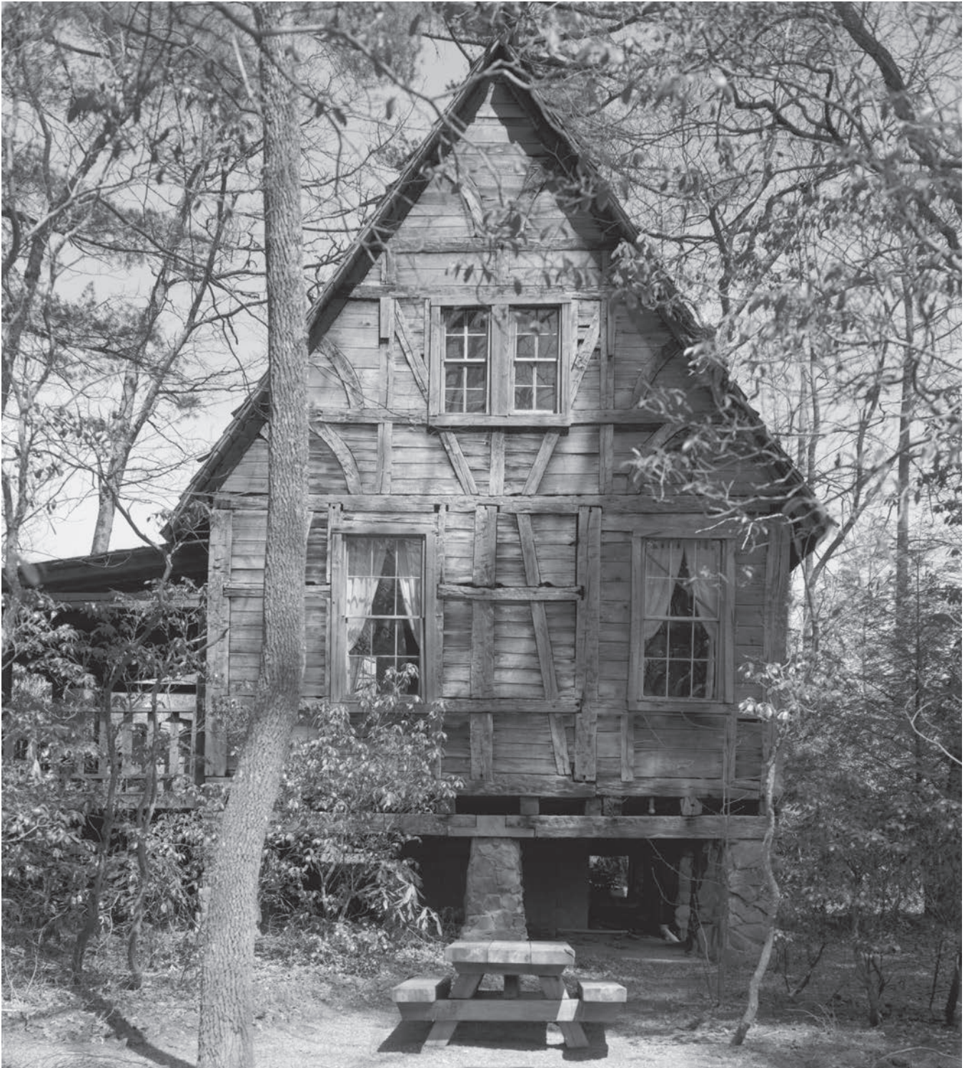
Image 14. Cantrell Creek Lodge, Biltmore Forestry School. (Source: Historic American Building Survey, loc.gov)
