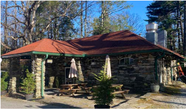
Image 58. This stone gas station in Caesars Head features rough-hewn stacked stone without visible mortar.
