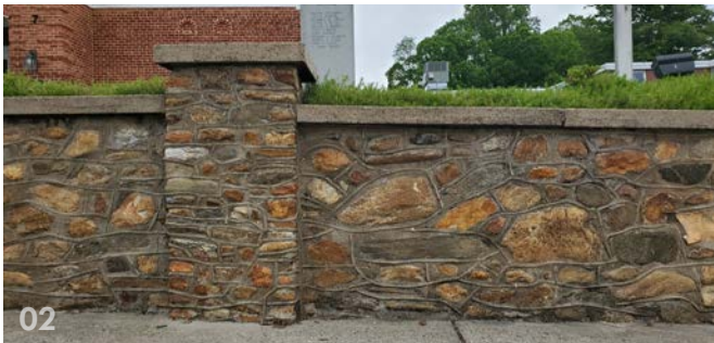
[01-02] Native stone retaining wall varieties in Downtown. [03] Hollingsworth Building wall draws on architectural concepts from the building.
