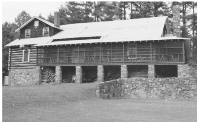
Image 27. Brevard Country Club, view showing stone foundation (Source: Digital NC)
