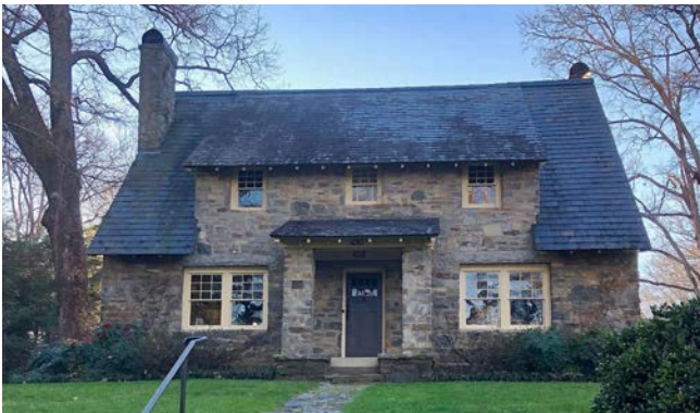
Image 60. The Royal and Louise Morrow residence is one of the oldest stone houses in Brevard, featuring coursed stone. (Source: Wikipedia)
