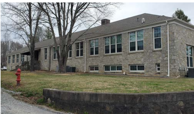
Image 62. The Rosenwald School, built with uncoursed native stone, grapevine mortar, and quoining at the corners.
