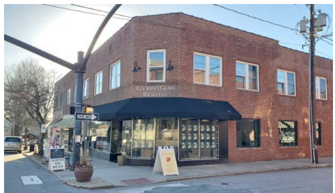
Image 46. Brick masonry vernacular building in Downtown.
