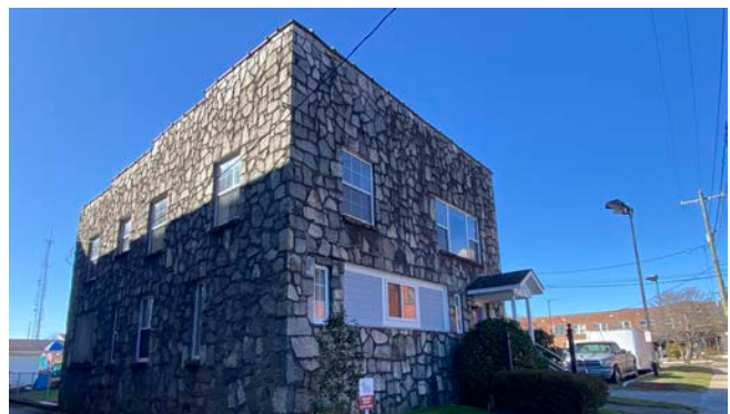
Image 57. Stone masonry vernacular building in Downtown at 134 Johnson Street, where stone is applied as a veneer .
