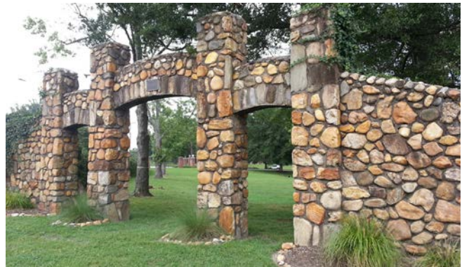
Image 54. Brevard College Stone Gate, built by local masons using stone from the Davidson River. (Source: Wikipedia)
