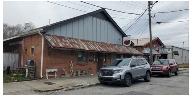
Image 74. Repurposed industrial building, the Lumberyard District.
