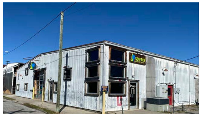
Image 75. Repurposed industrial building, the Lumberyard District.
