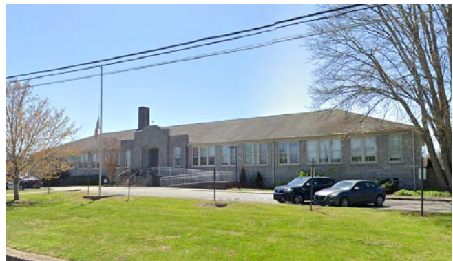
Image 55. Davidson River School, former Pisgah Forest School, built under the WPA using uncoursed stone. (Source: Google Streetview)
