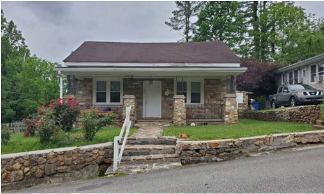
Image 103. Masonry house on West Ln, Rosenwald Neighborhood.
