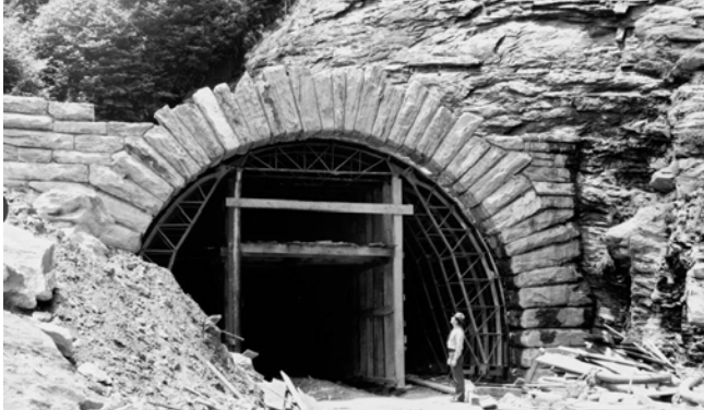
Image 25. Devils Courthouse Tunnel. (Source: Library of Congress)
